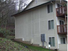
**DESCRIPTION:** The east side of building #628 shows an anomaly consistent with un insulated bays. The areas in question are at the location where the interior showers back up to the exterior wall. This could be the cause the anomaly, however no other buildings showed this type of anomaly. Non insulated bays may cause condensation within the wall.
