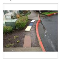
The walkways are variously damaged and should be repaired or replaced. The 2 entry steps are tiping down toward the building the same as building 606. The upper edge crack should be sealed and the situation monitered as with 606.
