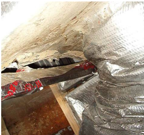
Figure 10. Large leak in return plenum at air handler
